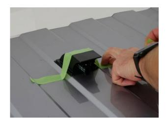
Remove the adhesive template and fix the roof duct
