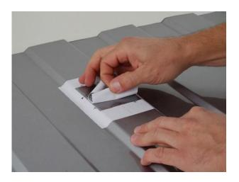
Remove chips and peel off the inner part of the sticker
